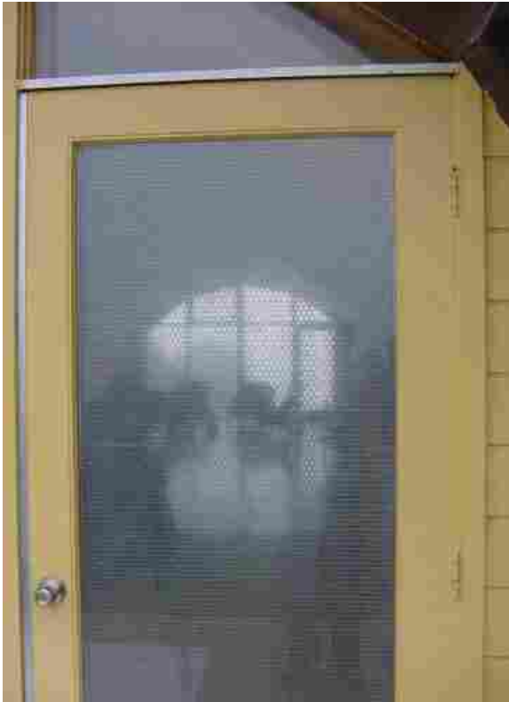
Fig 1. Visual performance of the bubble-glazed balcony door observed from outside. Interior details some 18m away are still recognizable. The bubbles have 10mm diameter and the bubble-wrap sheet is supported along the inside glass edges using aluminum channels.
