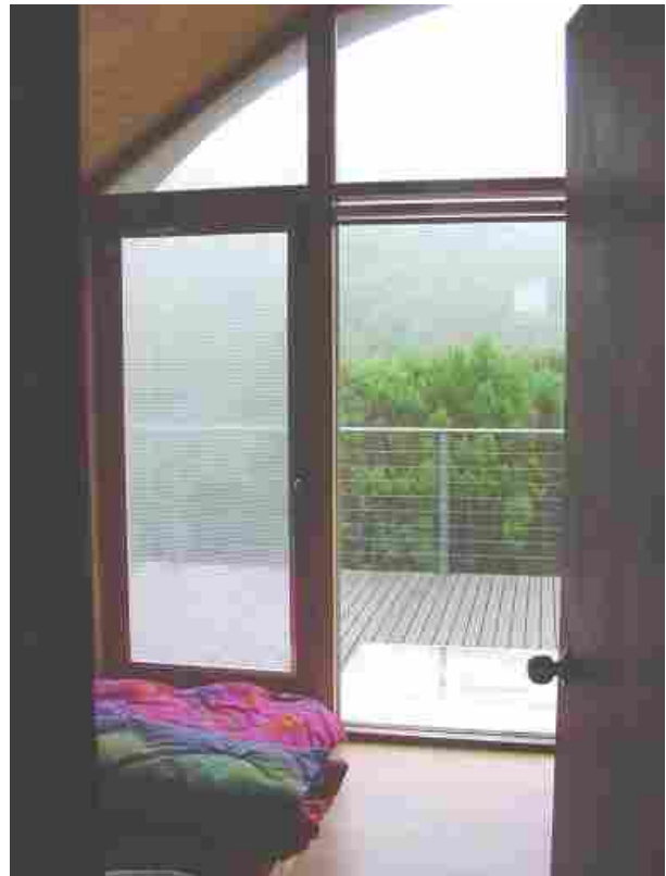
Fig 2. Bubble-glazed door in the southwestern bedroom window wall on a foggy winter day. It looks much like a frosted glass door, but its thermal performance is far superior. Unlike curtains, bubble-glazing transmits all incoming light that adds to the positive ambience of the room. Aluminum channels used to support the bubble-glazing do not reduce the size of the window. When bubble-glazing is removed for summer, aluminum channels will be stored in their best place: where they are needed in winter.
